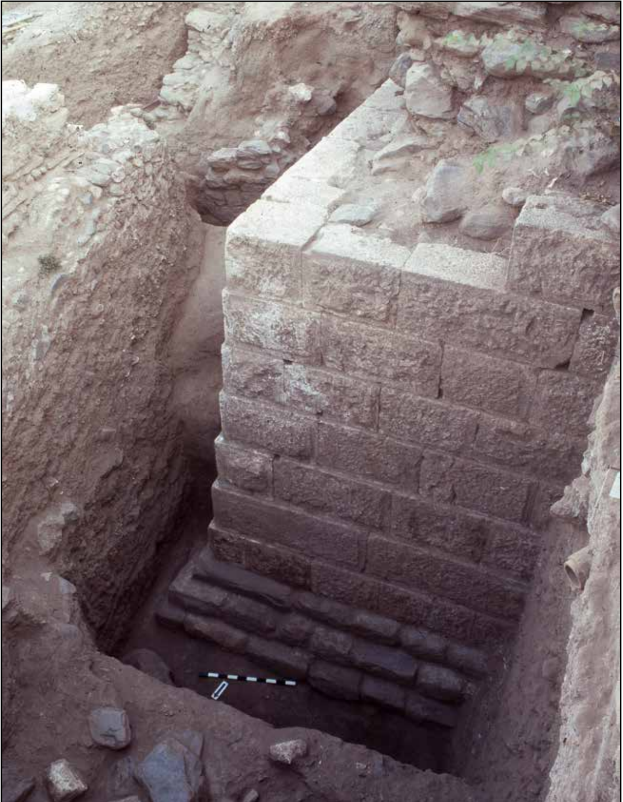
Figure 3: ByzFort, view of northeast corner (1985).
