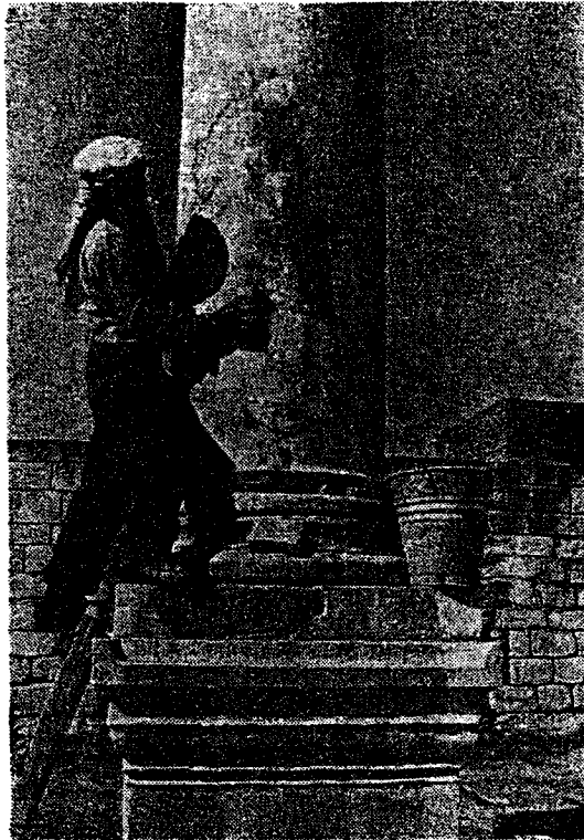
Fig. 3 Column in the southern colonnade of the Palaestra being cleaned (75)1.18
