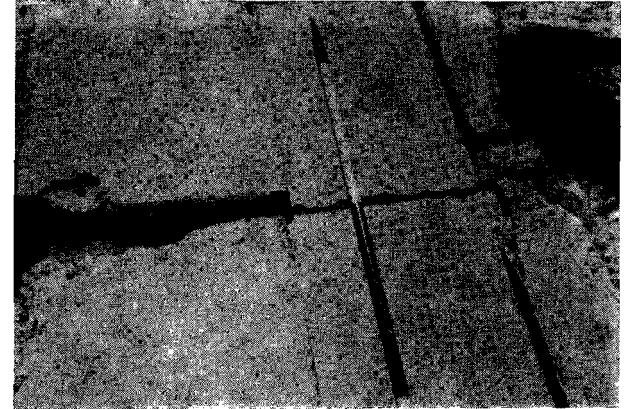
Fig. 6 - Detail of limestone base, remnants of clamps. Karaburun il.
