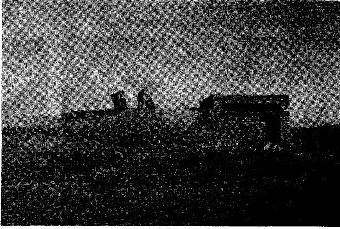
Fig. B- Kizilbel. *View of rebuilt Amulus and entrance building.
