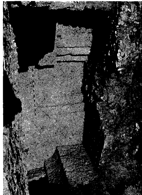
Fig. 12 — Anemurium: Exedra building (II 12 E), detail of facade wall, stylobate, and steps to west wing, seen from east.
