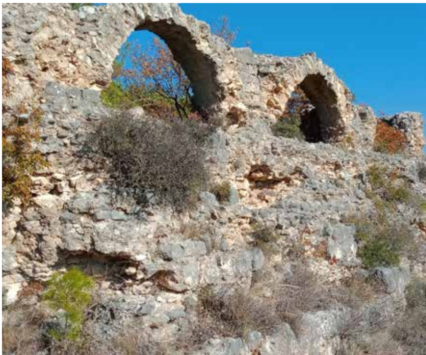
Figure 14: The Cistern at the End of the Third Waterway
